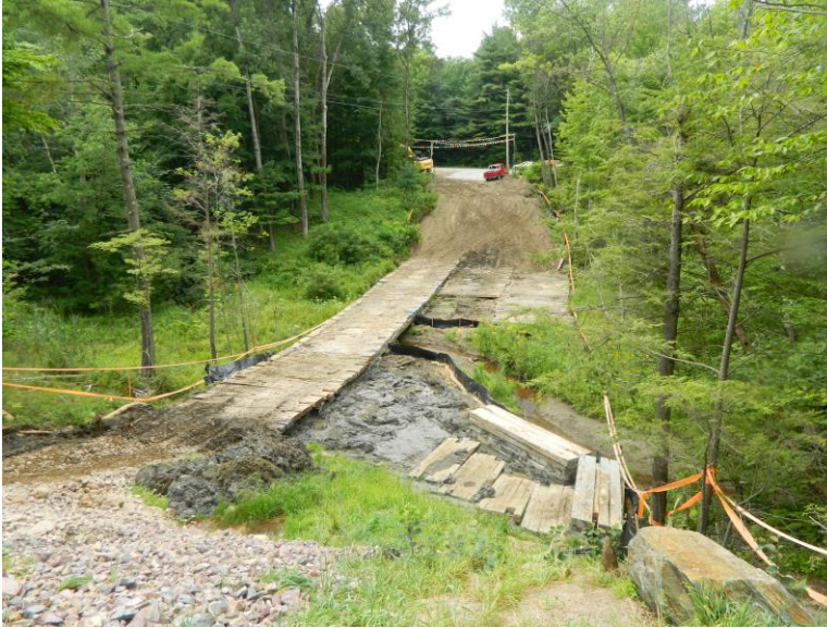
Photograph 1: Michels Pipeline Construction installing timber mats and access to Redmond Brook stream crossing. Matting also being installed in adjacent wetland 2012-CM-134.
