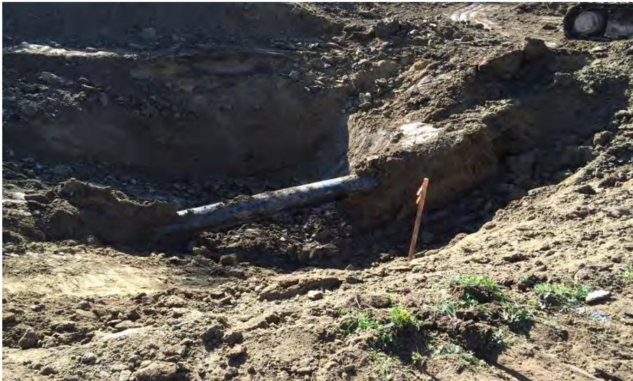
Exposed pipe section at station 565+85. Moved stake into area to show location of possible dent.
