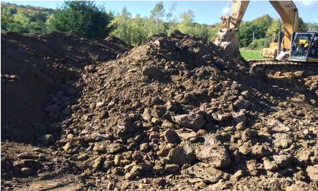
Excavation dirt pile with clumps of clay and no rocks. Expanded excavation to locate weld 0193.
