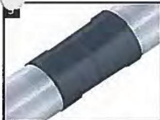
For heat-shrinkable sleeve corrosion coatings use the Canusa product specific installation guide.
