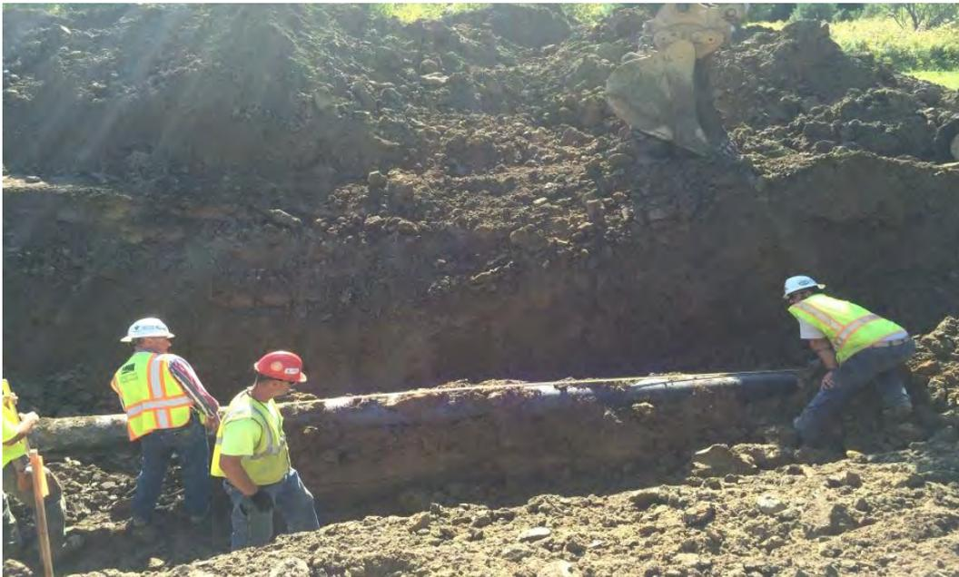
Measurement of 17' from weld 0193 to possible dent to confirm location.
